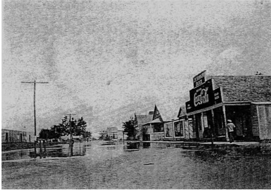
Figure 20: Floodwaters inundating downtown Morganza
