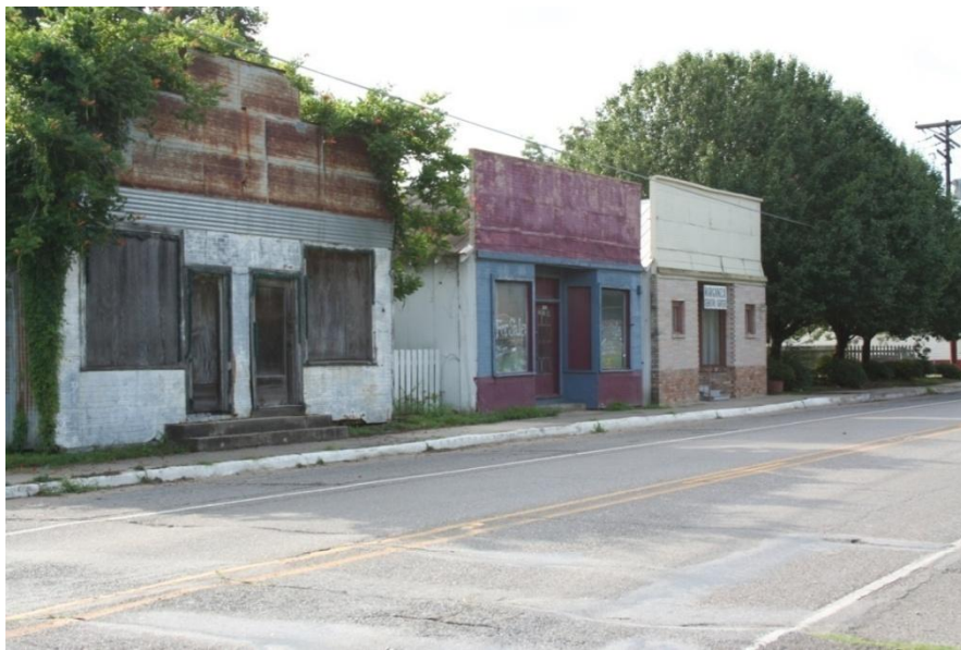
Figure 4: Abandoned buildings in downtown Morganza. Photographer is standing in front of the railroad dividing town
