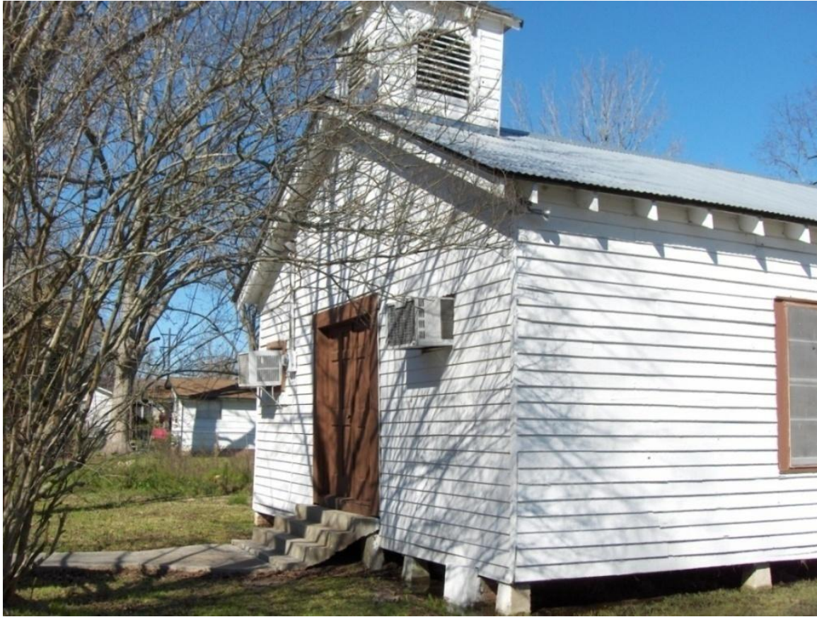
Figure 5: Starlight Baptist Church and footings
